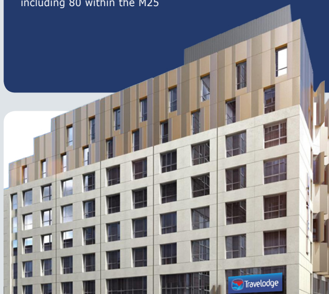
Our largest new build flagship hotel, close to the Gherkin, opening in 2018 395 rooms
